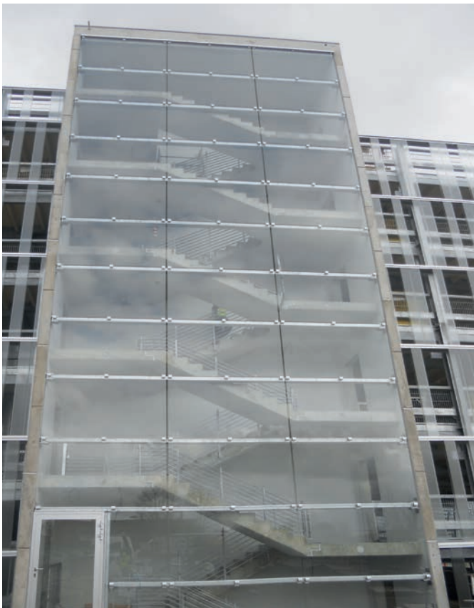
Parkhaus, Slough/Berkshire, England / Car park, Slough/Berkshire, UK
